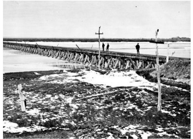
FIGURE 28 - WADES ON THE TRANSCONTINENTAL TELEGRAPH LINE AS IT CROSSES THE NORTH PLATTE RIVER IN NEBRASKA ADJACENT TO THE UPRR BRIDGE
