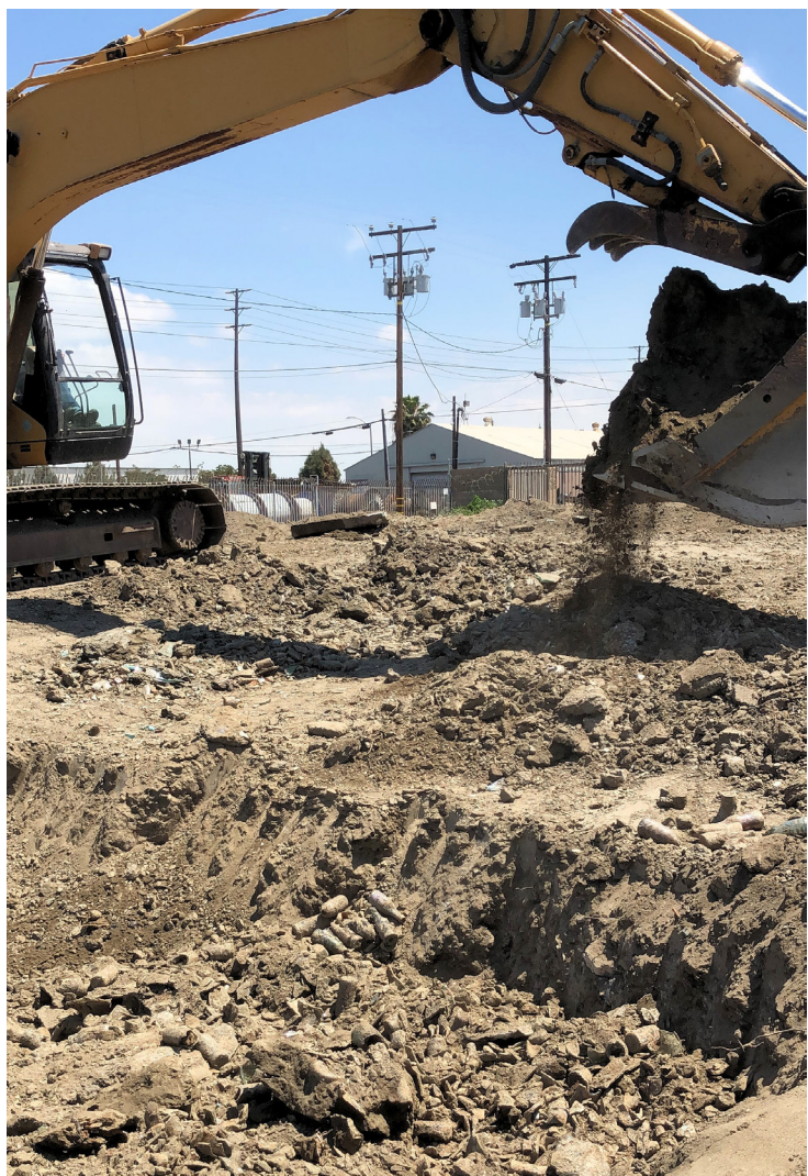
FIGURE 24 - THE EXCAVATOR EXPOSING THE CULLET LAYER
