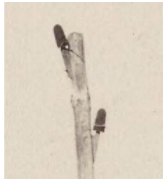
FIGURE 23 - (LEFT AND BELOW CENTER) ECHO CANYON TELEGRAPH STATION AND CLOSE-UP
