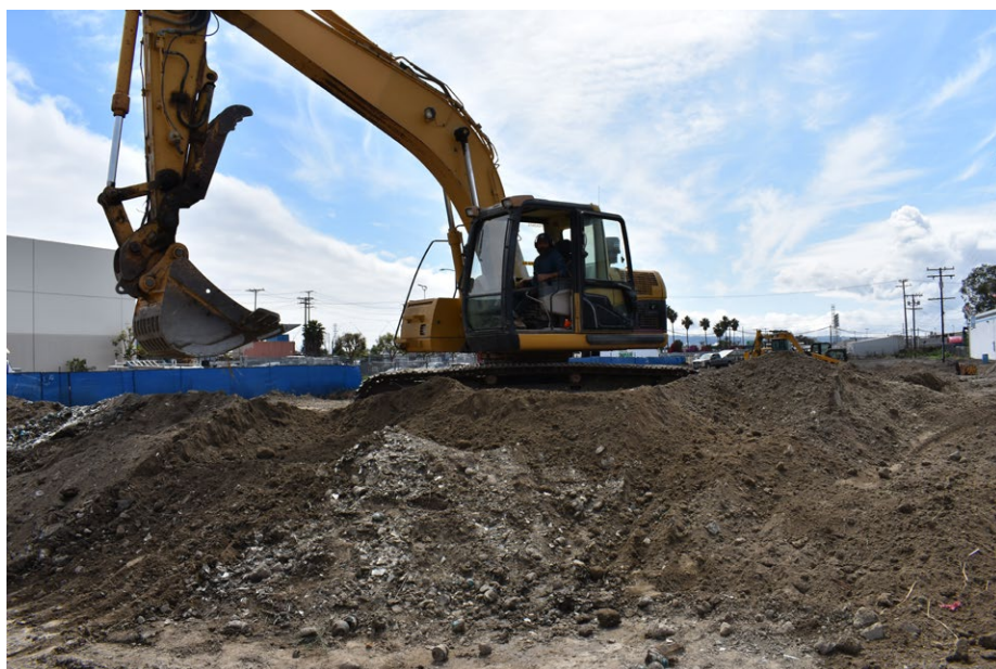
FIGURE 7: ASSISTANCE FROM THE EXCAVATOR
