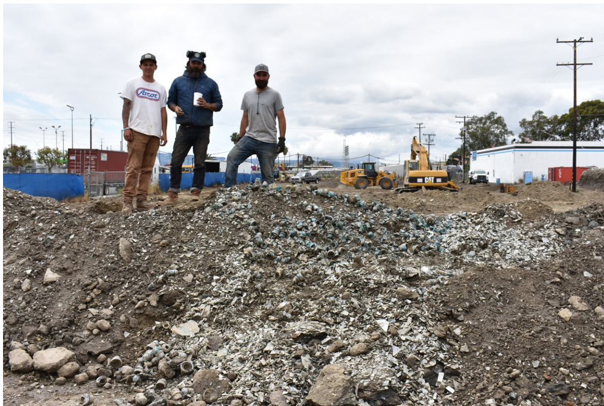
FIGURE 3: THE HEAVY EQUIPMENT WORK CREW
