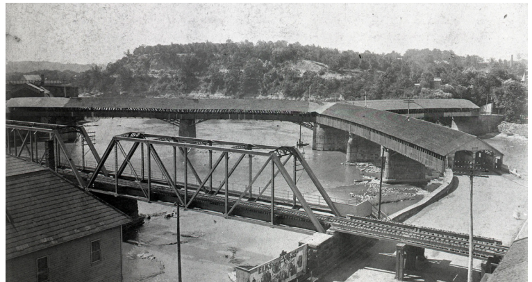
FIGURE 10 - THE 1832-1900 ZANESVILLE COVERED "Y" BRIDGE
