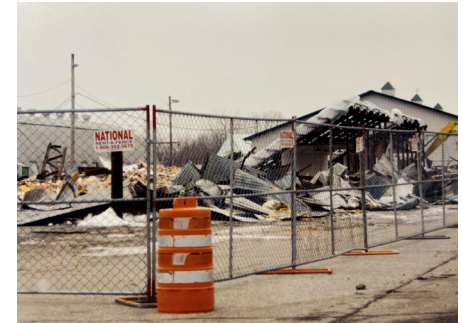
THE OLD QUONSET HUT IN PIECES
