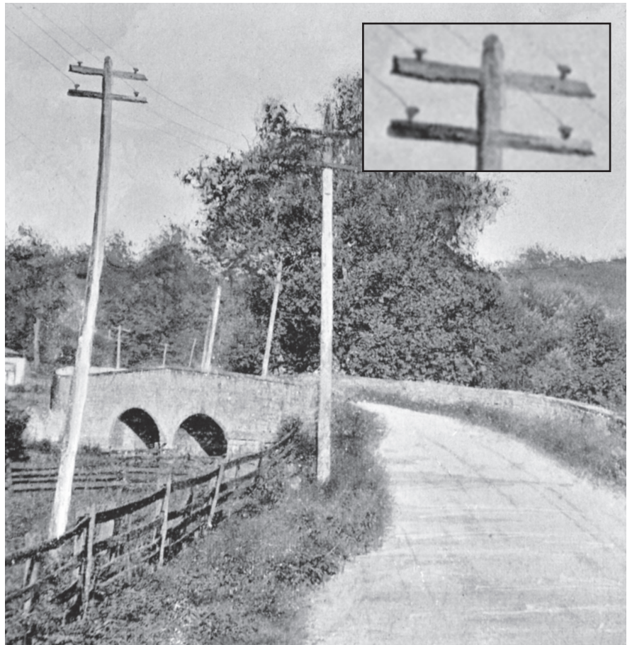
FIGURE 18 - AN EARLY PHOTO OF AN S-BRIDGE ON THE ROAD. WHILE THE SOURCE PHOTO IS LOW RESOLUTION, THE INSULATORS ON THE POLE TO THE LEFT CERTAINLY RESEMBLE SOME SORT OF "BUREAU KNOBS" (CLOSE-UP INSET)
