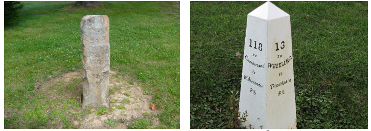
FIGURE 7 - AN ORIGINAL MILEMARKER AND AN 1835 REPLACEMENT replaced in 1835 by cast iron obelisk-type markers which were painted white with black lettering of the mileage and location information. (Figure 7) A few of the original markers remain.
