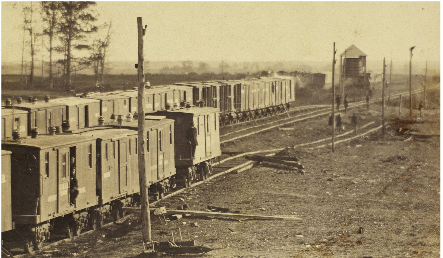
MANASSAS JUNCTION, VA IN MARCH 1864 - WHAT APPEARS TO BE A THREADLESS EGG ON THE TOP LINE WITH A WOOD BLOCK RAMSHORN MOUNTED BELOW ON THE OPPOSITE SIDE OF THE POLE (CLOSEUP RIGHT TOP)
