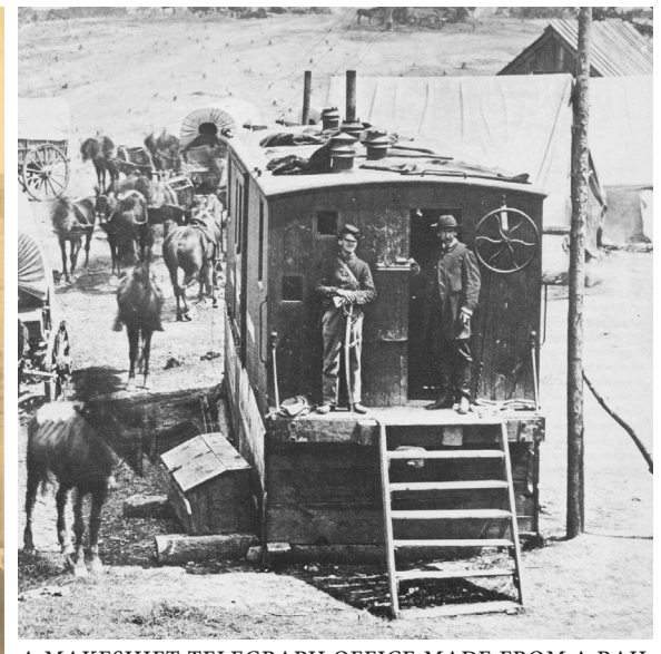
A MAKESHIFT TELEGRAPH OFFICE MADE FROM A RAIL CAR DURING THE CIVIL WAR - NOTE THE THREADLESS ON THE ROOF AT THE REAR LEFT OF THE CAR
