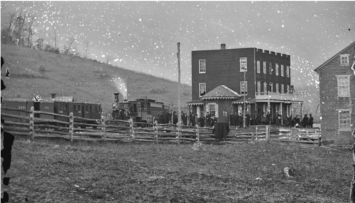
(ABOVE) HANOVER JUNCTION, PA. AS YOU LOOK CLOSELY AT THE PICTURE, USING YOUR INSULATOR SPOTTING EYES, SEVERAL THREADLESS ARE EVIDENT!
