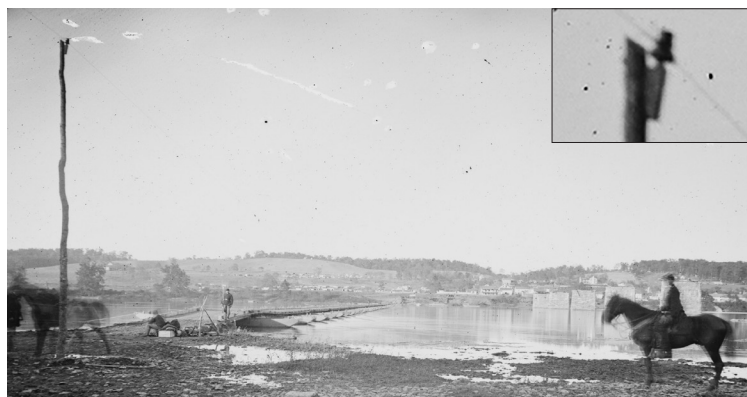
(LEFT) A SINGLE STOVEPIPE HAT THREADLESS SUPPORTS THE WIRE AT THE END OF THE UNION ARMY'S PONTOON BRIDGE OVER THE POTOMAC RIVER AT BARRY, MARYLAND (NOW BRUNSWICK). CLOSE UP IMAGE INSET.
