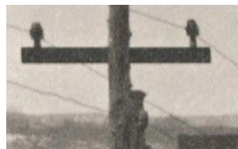
OUT WEST AFTER THE CIVIL WAR, WE SEE THREADLESS IN USE ON THE UNION PACIFIC.
