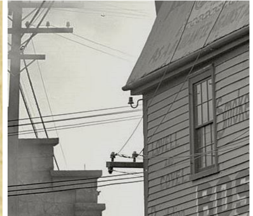
ONE OF MY FAVORITES. THE 737 STOVEPIPE HAT REALLY STANDS OUT ON THE NICE FORGED STEEL BRACKET MADE WITH A CURVE ON IT. LIKELY TO BE IN BOSTON
