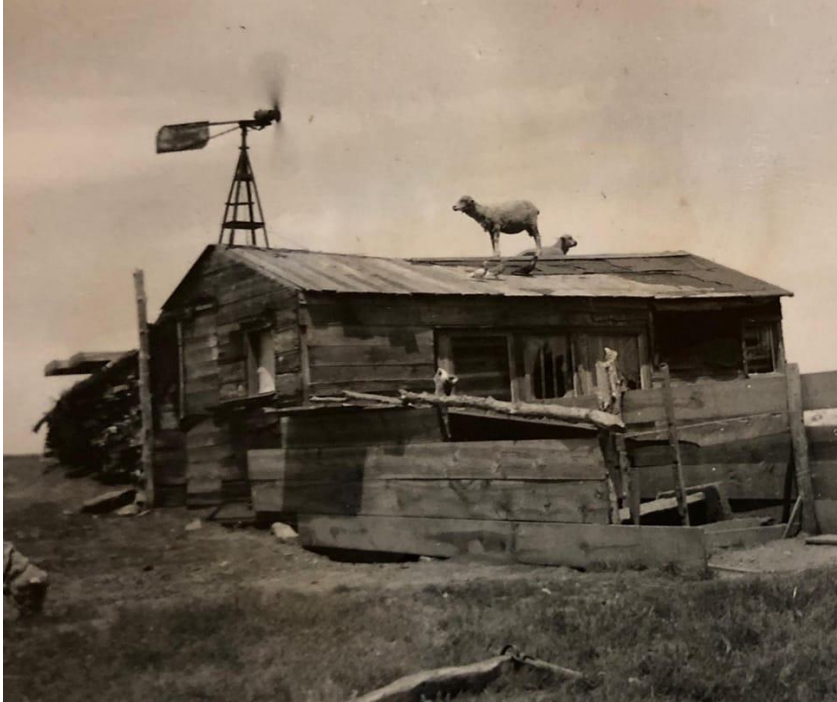
17.1.2 shows a 6-volt Wincharger mounted on a rooftop.
