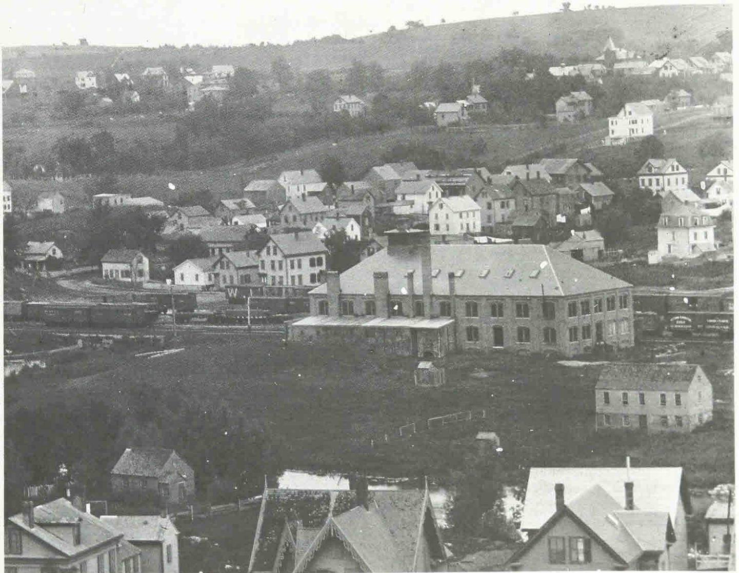
(Figure 1.) 1888 photograph of the American Iron Glass Pipe and Plate Company plant in Haverhill, Massachusetts. (Photo is courtesy of the Haverhill, Massachusetts, Public Library)
