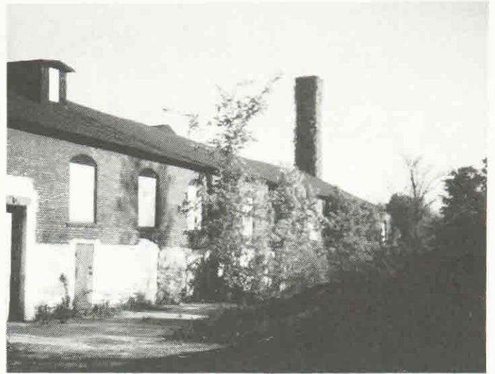
Another part of the abandoned factory which formerly housed the Ohio Valley Glass Company. (Photo courtesy of Bob Harding)
