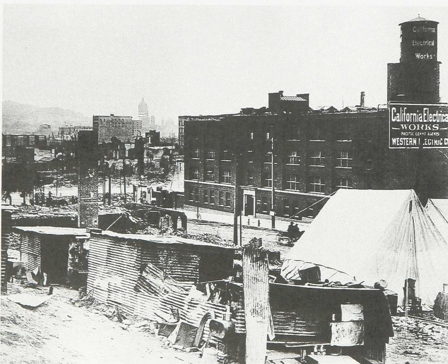
(Figure 7.) The 642 Folsom Street plant of California Electrical Works. Note that the sign on the building indicates that they are the West Coast agents for the Western Electric Company. (Photo by Hans Kettenburg from Ron Ross collection, courtesy of Glenn Yows)
