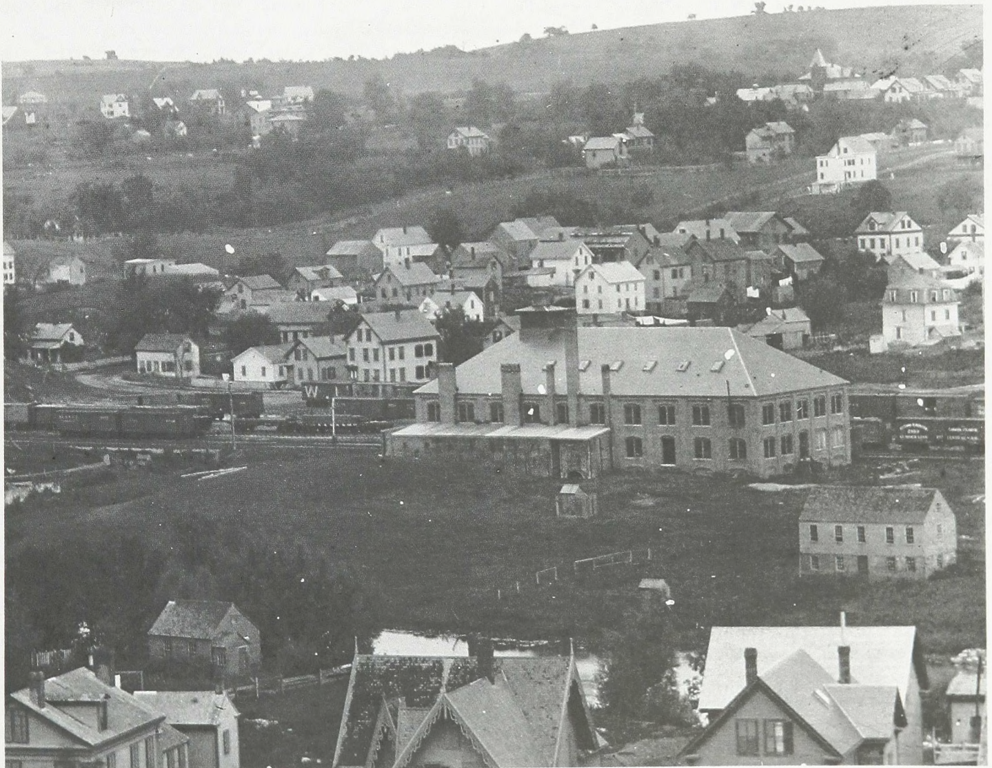
(Figure 1.) 1888 photograph of the American Iron Glass Pipe and Plate Company plant in Haverhill, Massachusetts. (Photo is courtesy of the Haverhill, Massachusetts, Public Library)
