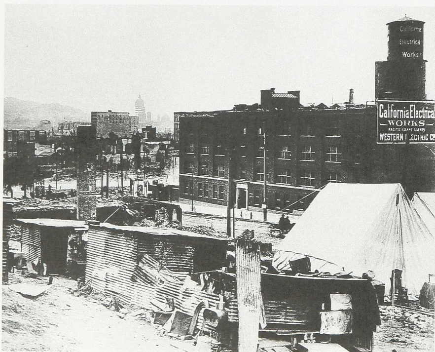
(Figure 7.) The 642 Folsom Street plant of California Electrical Works. Note that the sign on the building indicates that they are the West Coast agents for the Western Electric Company. (Photo by Hans Kettenburg from Ron Ross collection, courtesy of Glenn Yows)
