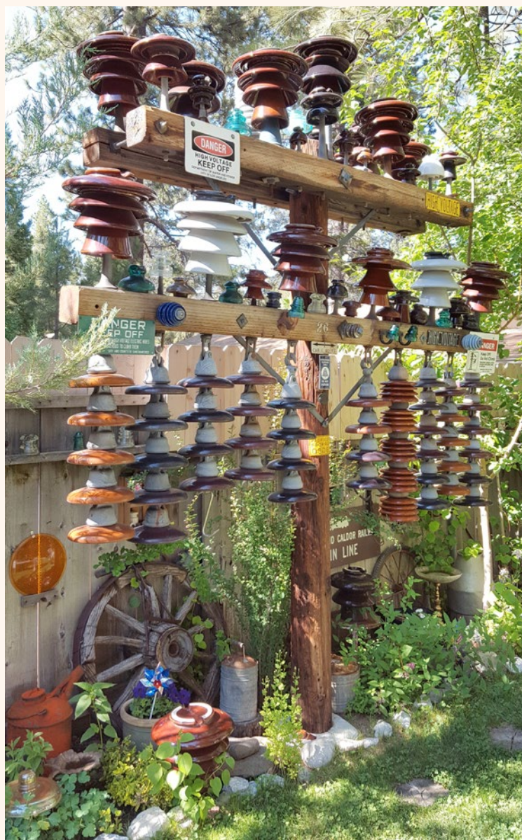
One of many towering, spectacular High Voltage hardware exhibits in the back yard.
