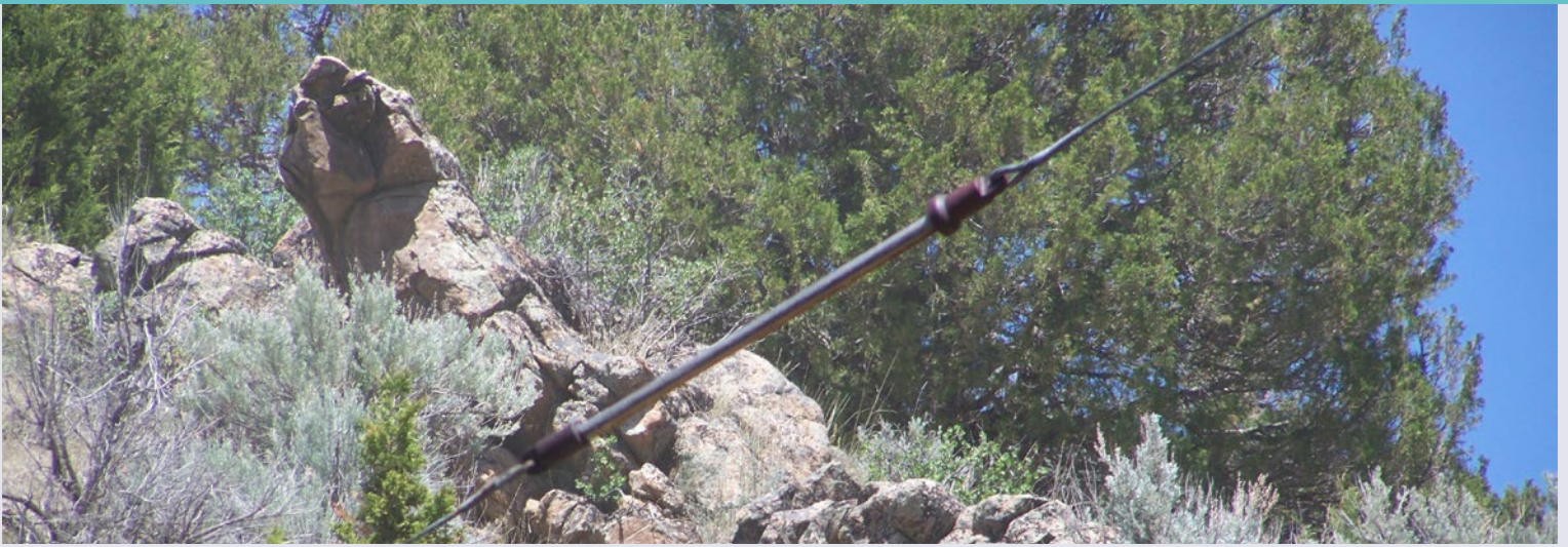
Most of the pins for the small 10 bell sets were used as guy wire insulators.
