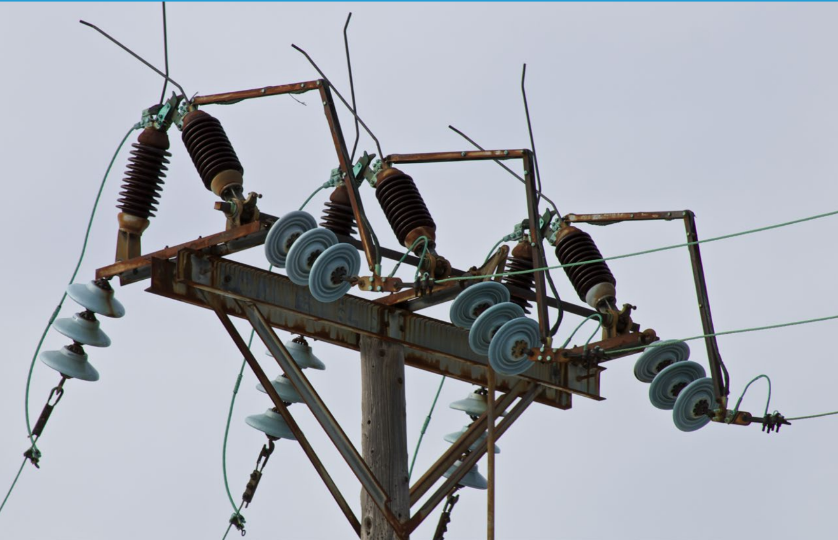
Blue J-D ST-6800 Discs in use in a old substation in Michigan | Photo by: Shaun Kotlarsky
