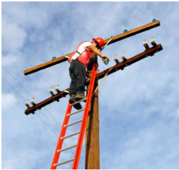
Above an example of a pole with 5 Smooth Base McLaughlin insulators on it.
