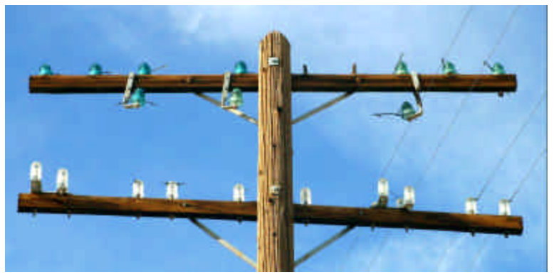
Above an example of a pole with 5 Smooth Base McLaughlin insulators on it.
