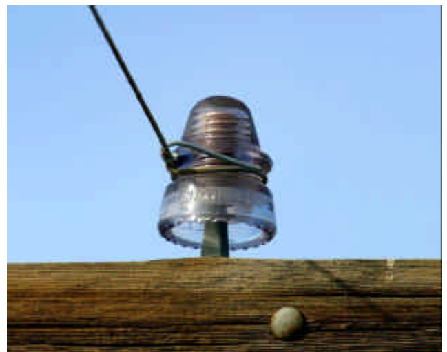
Above left, can be seen a pole bearing two purple tinted Maydwell 19's. At right, a closer view of one of the Maydwell's
