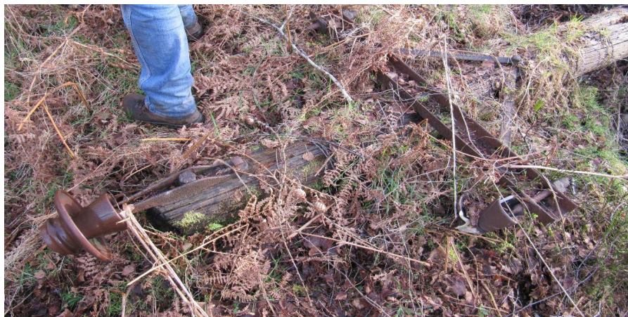
LEFT: PHOTO 6 – THE FALLEN POLE WITH TWO UMBRELLA PATTERNS STILL IN PLACE
