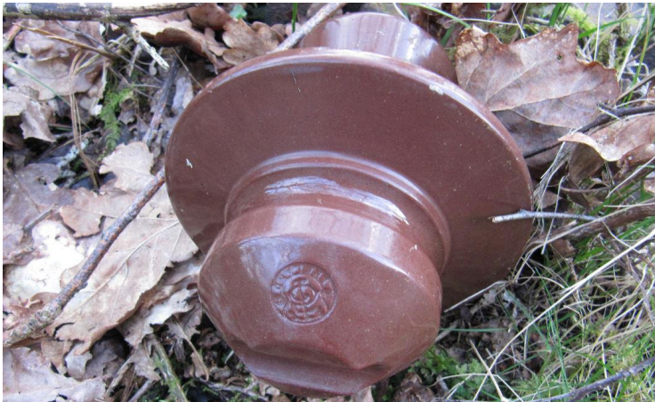
ABOVE: PHOTOS 11&12 – EARLY TTC DELTA ON DISCARDED CROSSARM & ANOTHER POLE FOUND FURTHER ALONG CONTAINING SMALL WHITE DELTAS.
