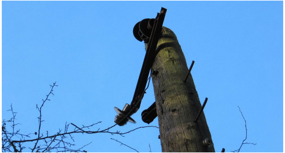
ABOVE: PHOTO 4 – THE ORIGINAL SURVIVING POLE CONTAINING THREE 'UMBRELLA PATTERN' INSULATORS.
